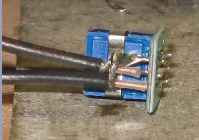
the two coax cables share a common ground
