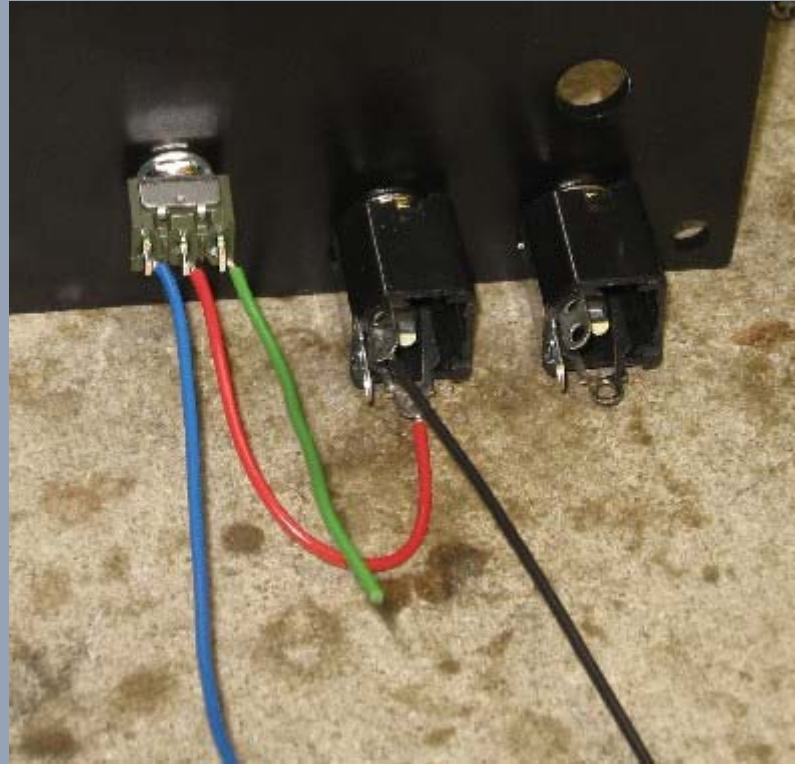
a 3in. bit of wire for the MIXED OUT jack shank lug so we can take ground from the OUT 3 jack
